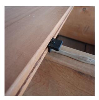
Once you've installed clips on every joist along the edge of the first board, slip the leading edge of the 2<sup>nd</sup> board into the clips snuggly.
